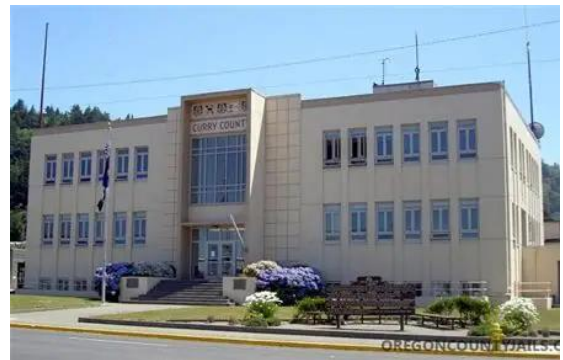
Figure 9: Curry County Courthouse, Gold Beach
