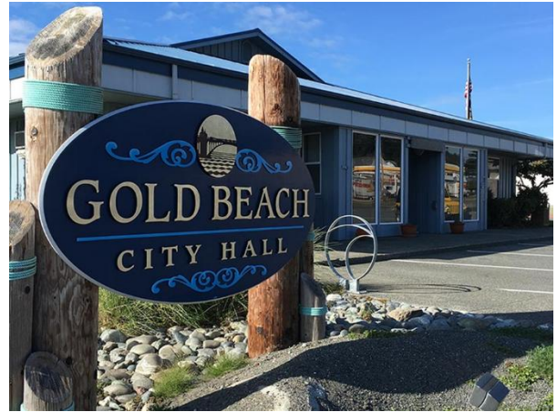
Figure 8: Gold Beach City Hall/Police Station
